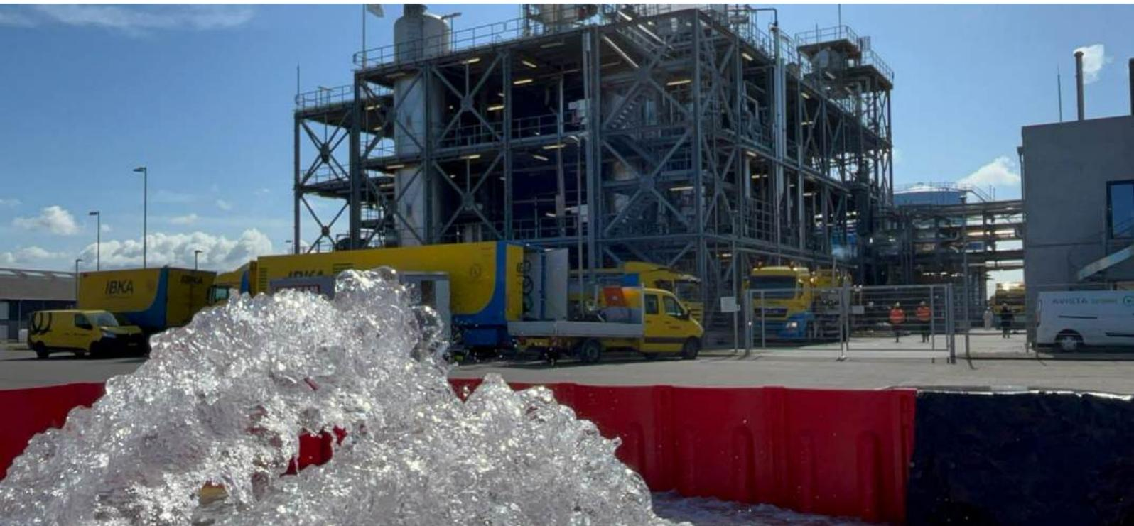
No additional tools are required for installation. However, in windy conditions, additional ballast can be placed at the base of each barrier module for stability until the floodwater anchors it. Furthermore, the stackable design of the NoFloods BoxWall facilitates efficient transportation and storage, minimising space requirements.
